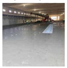
4000 PSI Well Graded Mixes were used for all interior slab on grade placements and 4000 PSI mix for all footings, foundation walls, stoops, and aprons. The admixture package also included a high range water reducer to help with workability and paste volume for coating the fiber strands. The project incorporated heated floors and intricate vehicle bays placements so cleaning and working under vehicles has easy access.
